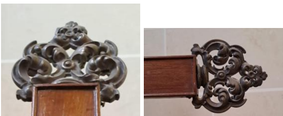
Figure 13: Two of the three finials of another crucifix. Cleaning tests should be undertaken to determine if they need re-plating.
