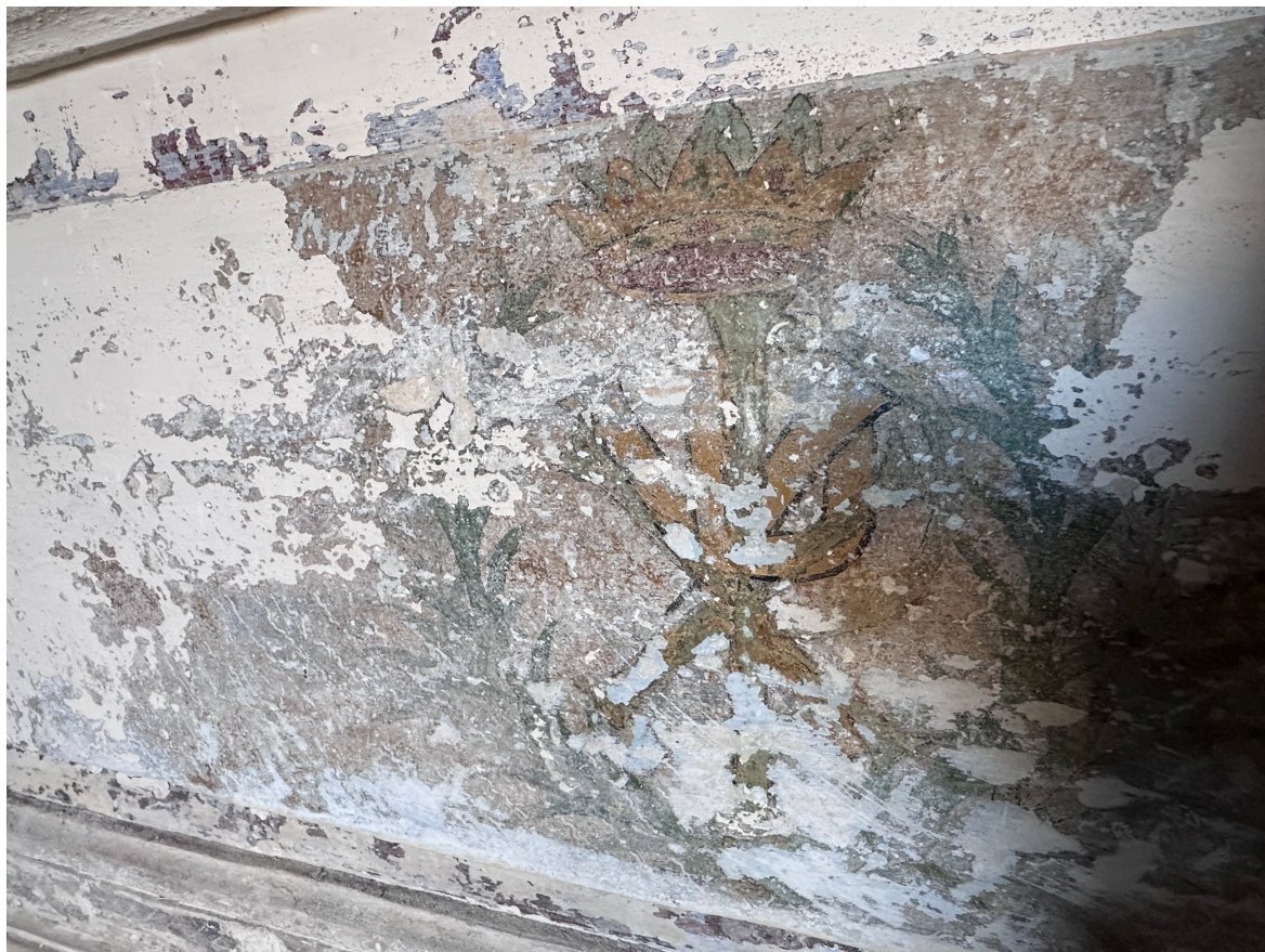
Figure 6. Powdering and faded oil colours. (Image, Restawr Arti, 2025)
