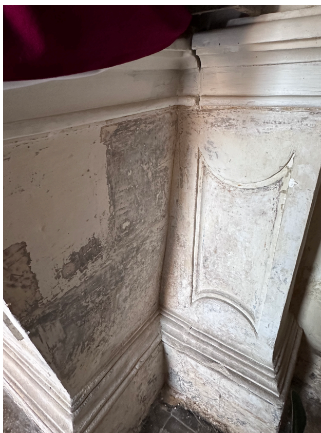
Figure 7. Lost painted decoration and exposed stone support. (Image, Restawr Arti, 2025)
