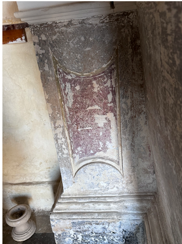
Figure 4. Original 19th century finto marmo exposed due to the natural deterioration of the re painted surface, and a previous restoration intervention. (Image, Restawr Arti, 2025)
