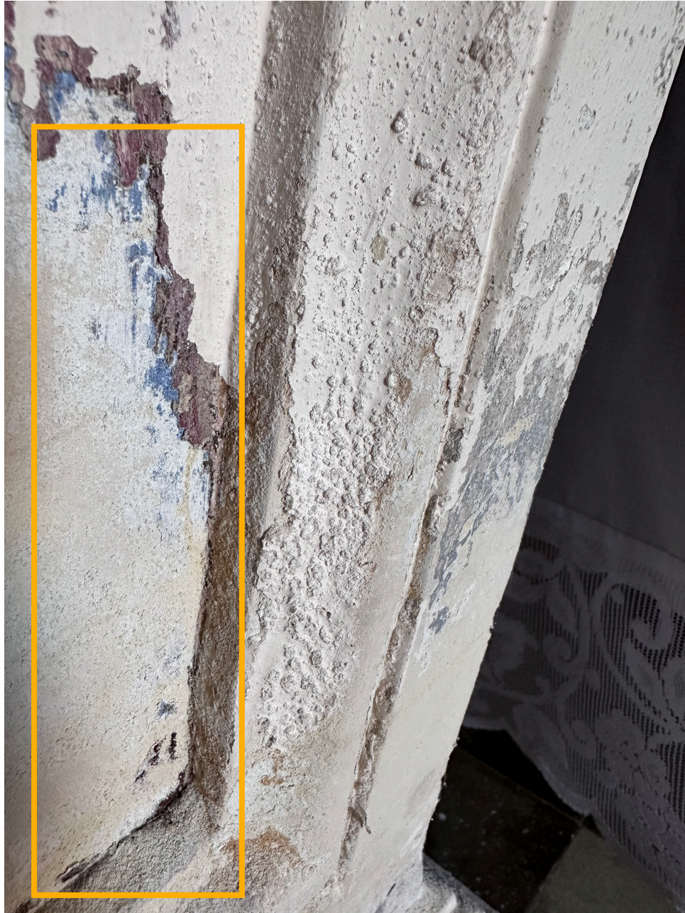
Figure 8. Stone powdering and salt efflorescence. (Image, Restawr Arti, 2025)
