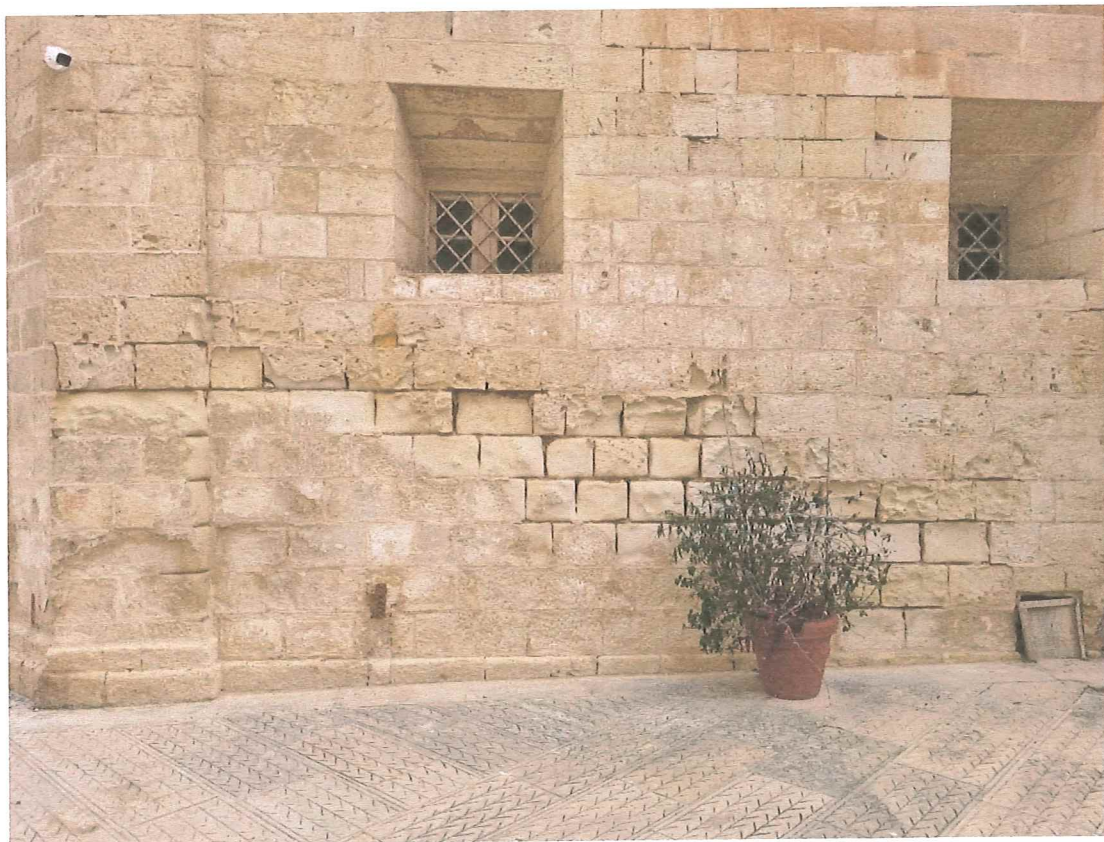
Image 05 – Area showing deteriorated stone which will require stone replacement and plastic repair, apart from raking of joints and re-pointing
