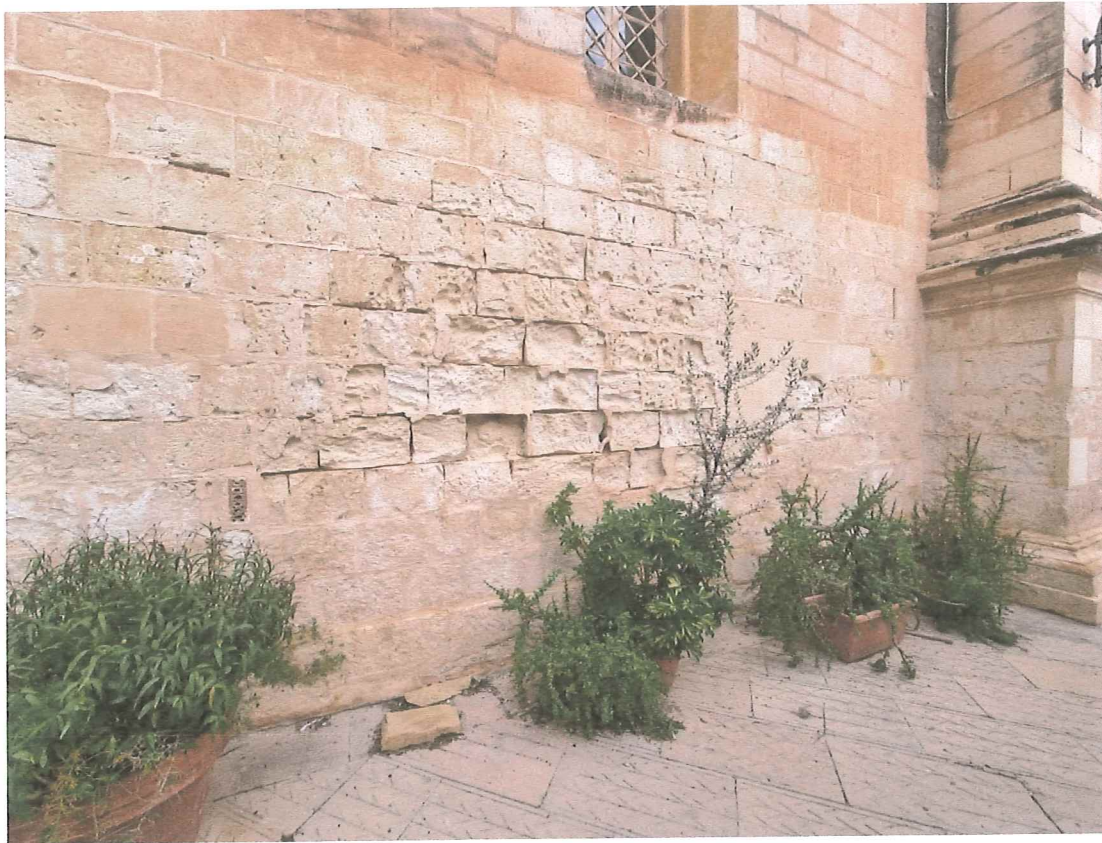
Image 04 – Area showing deteriorated stone which will require stone replacement and plastic repair, apart from raking of joints and re-pointing
