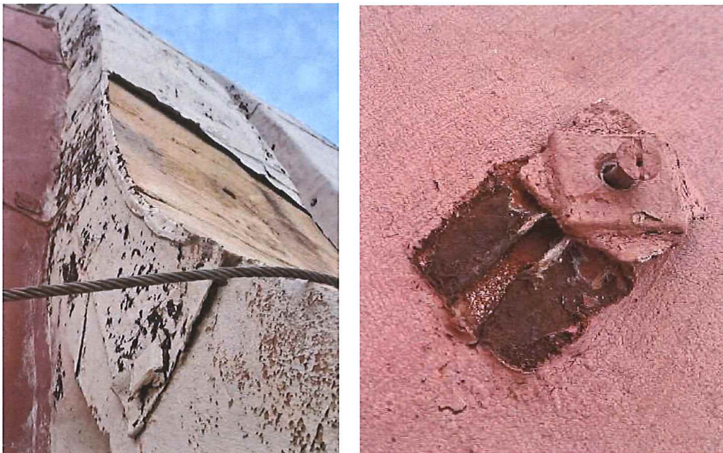
Figure 4-7 – missing lead sheets and slotted hole created by cyclic movement of the lead sheet relative to the fixture and the masonry.
