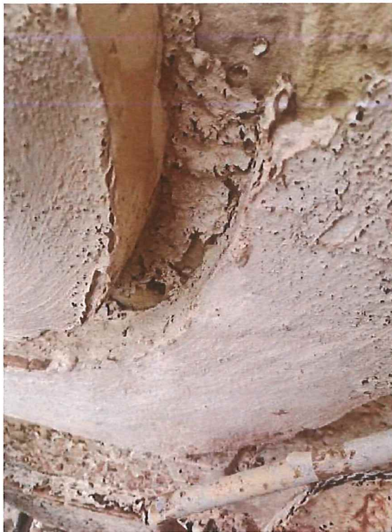
Figure 0-2 – Exfoliating white paint, vegetal deposits, paint deposits at preferential zones showing possible water entrapment.
