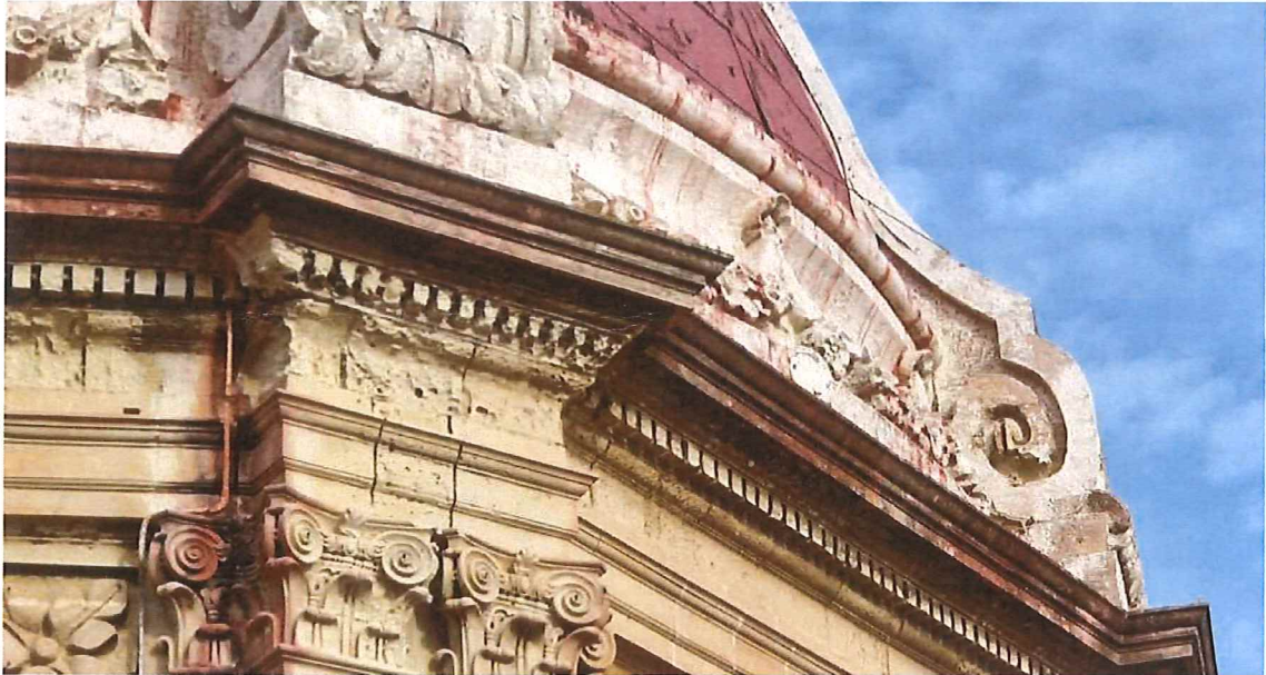
Figure 4-3 – Weathering and deterioration of the frieze below the main cornice of the drum.
