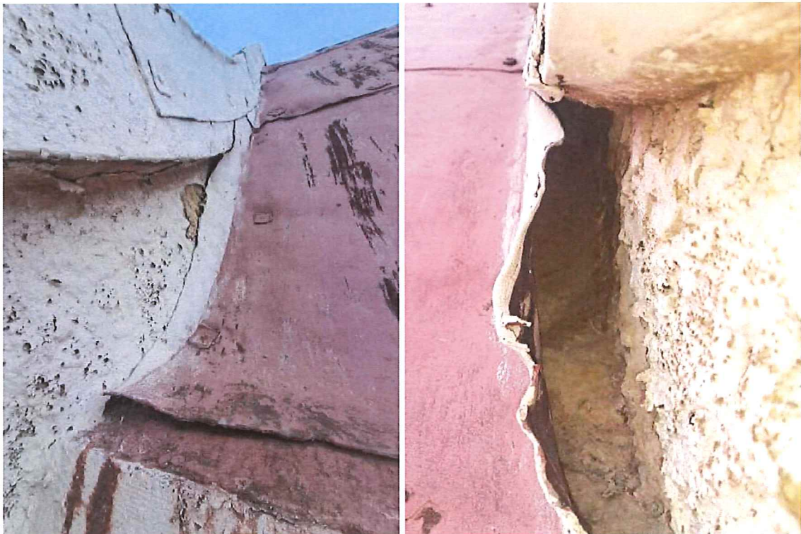
Figure 0-3 – Delaminating and detachable lead sheets used as waterproofing.
