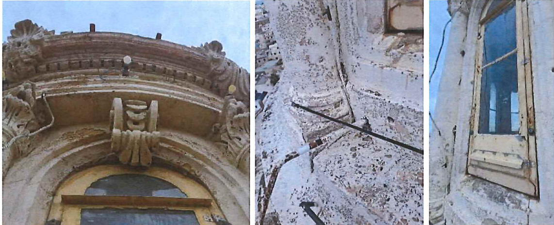
Figure 4-8 – closeups of masonry mouldings at lantern level showing deterioration and flaking protective paintwork
