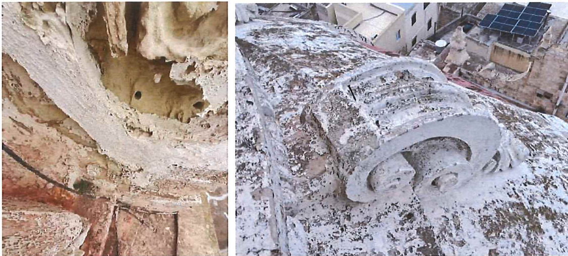
Figure 4-5 – weathering of the paint system, exposing the underlying masonry
